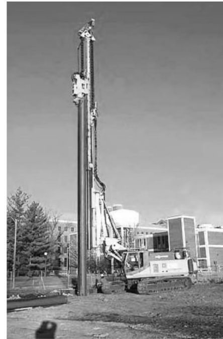
Figure 3.1 ABI Mobilram with telescopic leader fully extended driving tubular pile (courtesy ABI GmbH).
